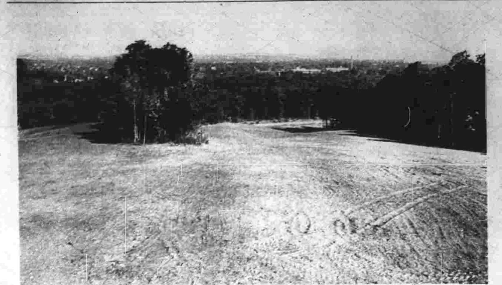
The new, 1,000-foot, six-lane dam on the south side of Hercules Dr. near the Mile Hill water tower for power, lights, and snow according to William O'Neill, public works director.
