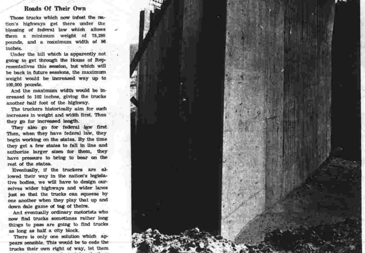
ROUTE 6 ABUTMENT Photographed by Reginald Pinto
